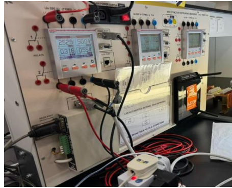
Figure 5. Measurement setup showing ATEMS validation against Lovato DMG800 power multimeter
