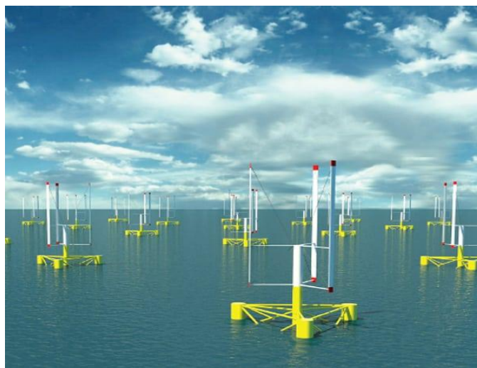
14-rasm. Vertiwind. Frantsiyaning Technip kompaniyasi va hamkorlari Nénuphar va EDF Energies Nouvelles, shu jumladan, Darrieus H-rotor dizaynini dengizda sinovdan o'tkazadigan loyihani boshladilar.
