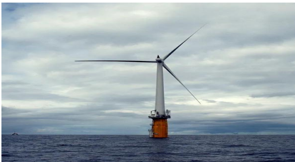
8-rasm. Birinchi to'liq miqyosli suzuvchi shamol turbinasi (2.3 MW)( Hywind Prototype (2009) )
