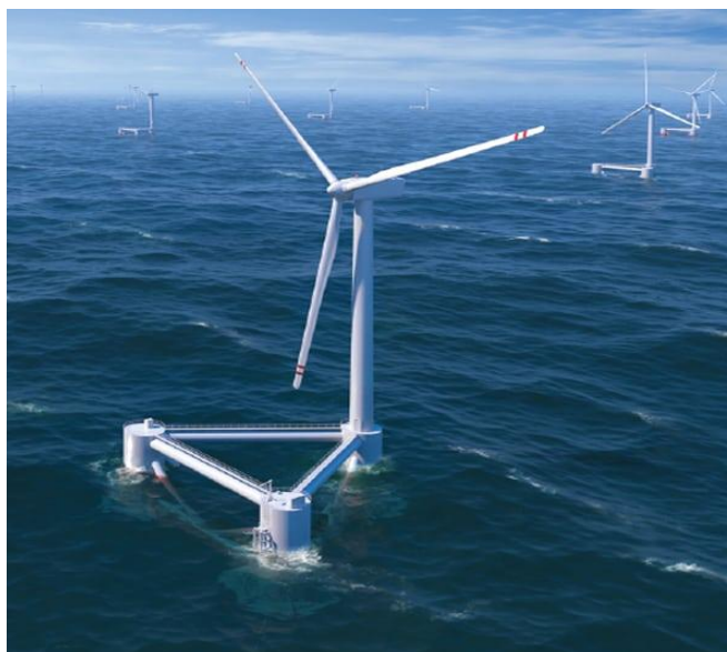
10-rasm. Portugaliya sohilida 2 MVt quvvatga ega suzuvchi shamol turbinasi
