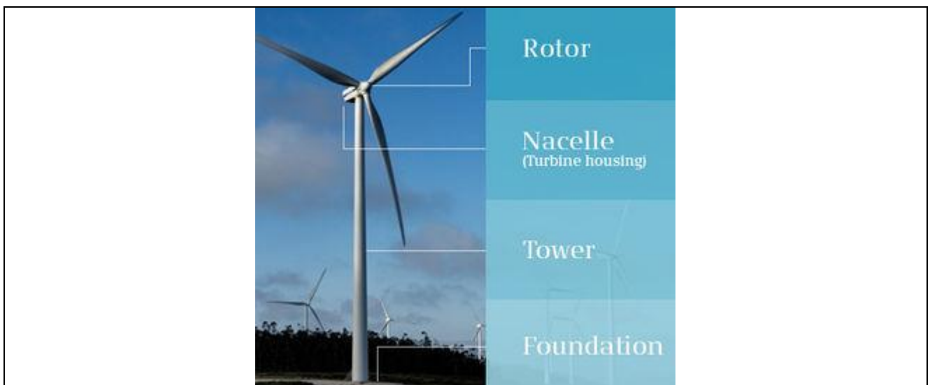
Figure 39. Construction of Wind turbine
