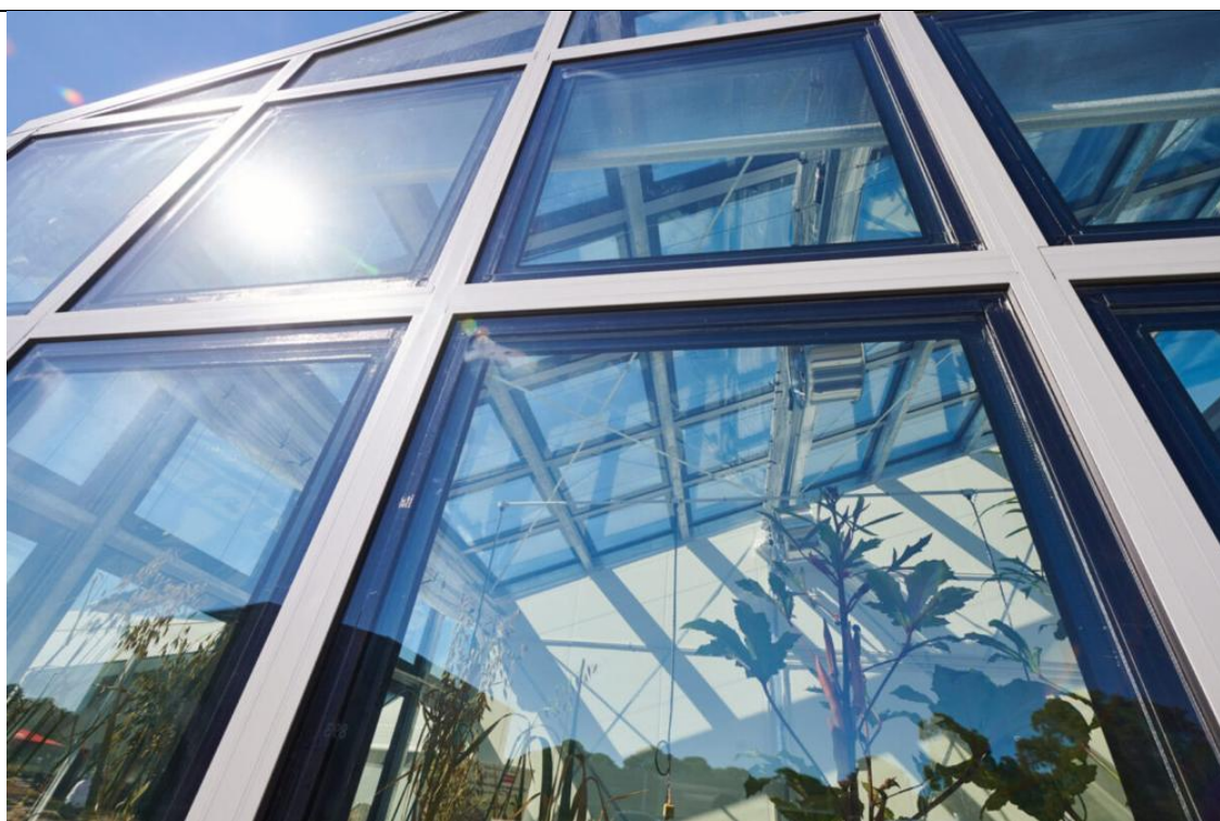
Figure 13: A greenhouse installation using ClearVue transparent solar windows. The glass panels (seen in the walls and roof) look nearly identical to conventional glass, maintaining about 70% transparency, yet they contain an integrated photovoltaic function that generates electricity from sunlight[24]. In this two-year trial at Murdoch University, Australia, the solar windows produced \sim 30 \text{ W/m}^2 and powered fans and environmental controls, while allowing sufficient light for plant growth. This showcases the application of transparent PV in agriculture, where it provides both shelter and energy without significantly impeding the sunlight needed by crops.
