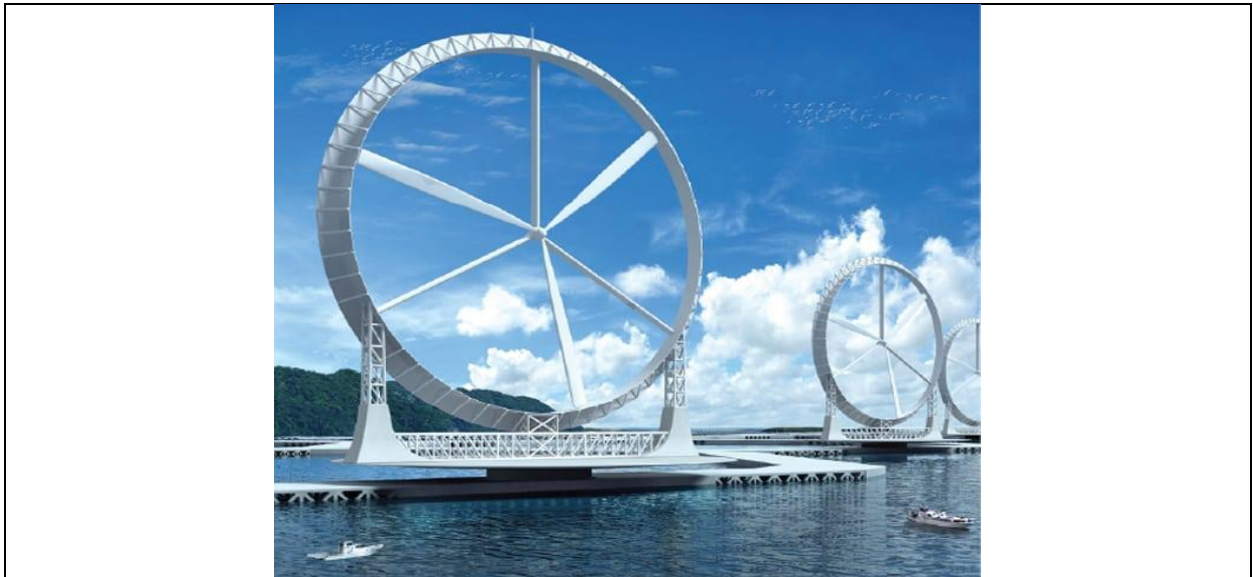
Figure 11. The Wind Lens. The shrouded horizontal-axis wind turbine for offshore use
