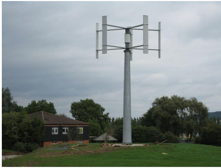
Figure 27. VAWT – Vertical Axis Wind Turbines. Savonius is another type of VAWT
