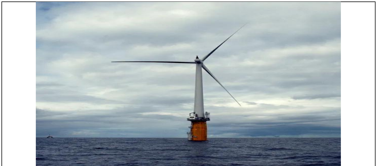
Figure 8. First full-scale floating wind turbine (2.3 MW)(Hywind Prototype (2009))
