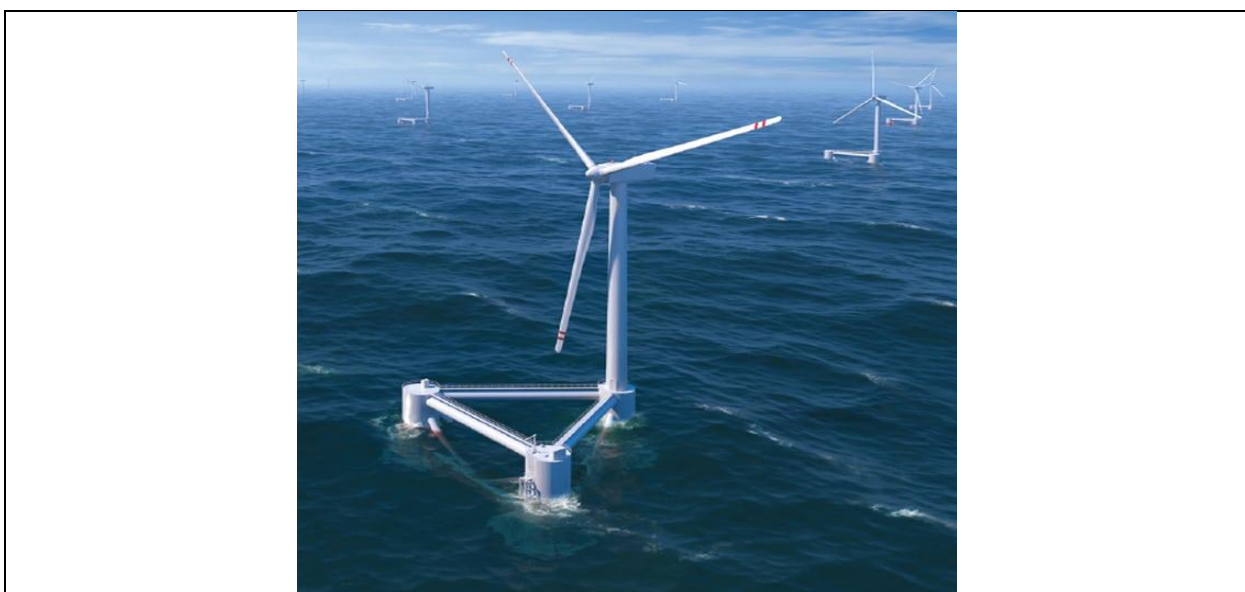
Figure 10. 2-MW floating wind turbine off the Portuguese coast
