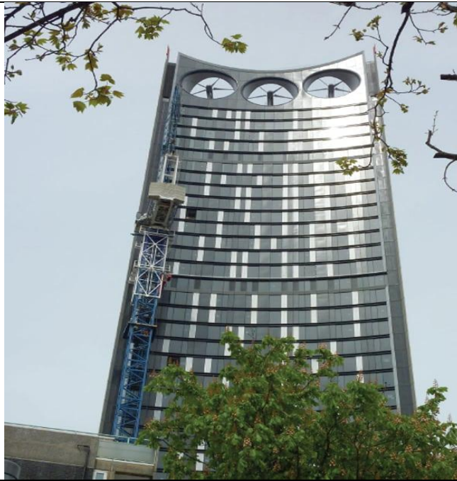
Figure 23. Tower of London. The Strata Tower in London’s Elephant and Castle neighborhood is a 43-story, 147-meter-high building that features three five-bladed built-in wind turbines.
