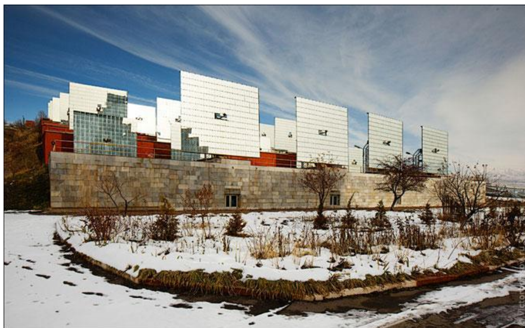
Figure-3.3.10. General view of the Large Solar Furnace and its heliostat field (Parkent district, Tashkent region).
