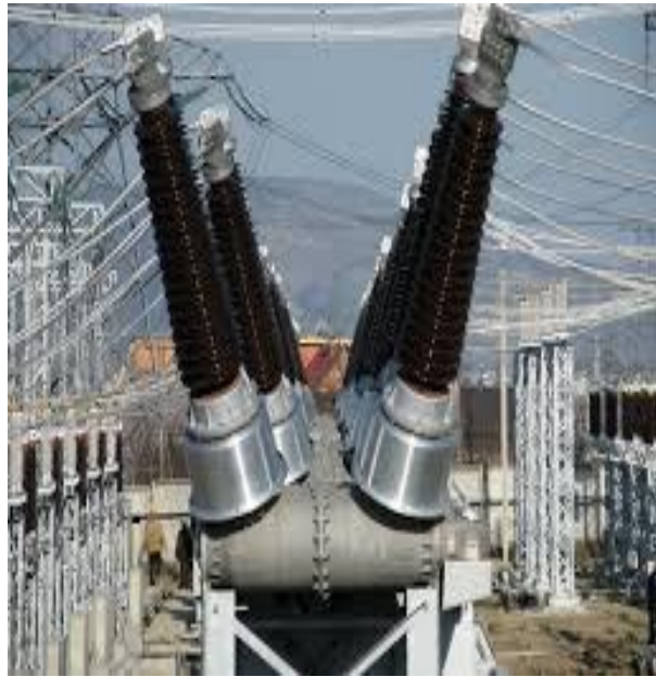
Figure 62. Gas-insulated circuit breaker used in high-voltage networks.
