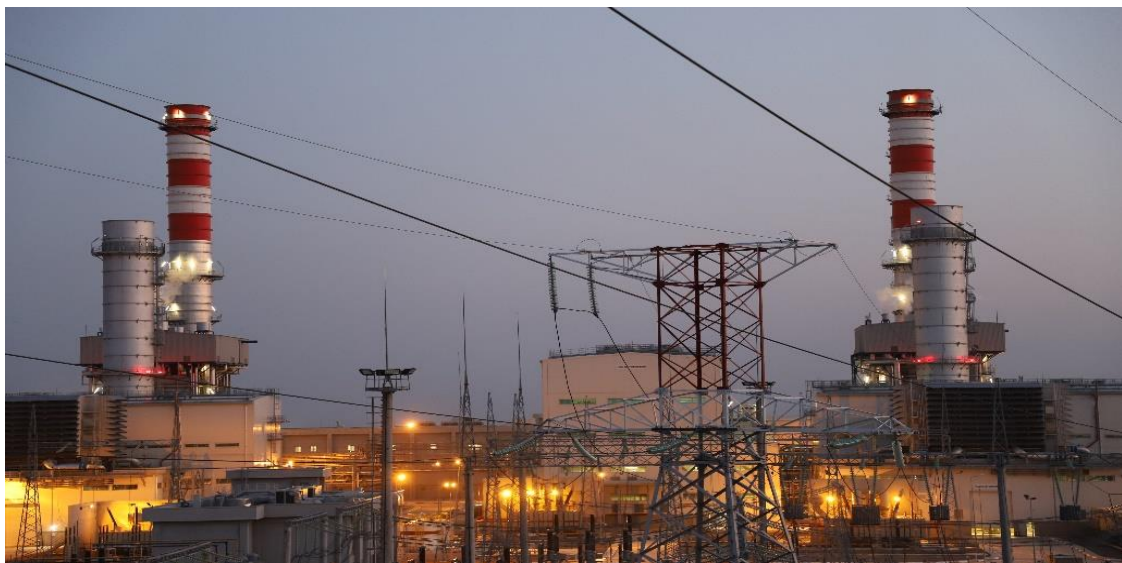
Figure 1. Thermal power plant.
