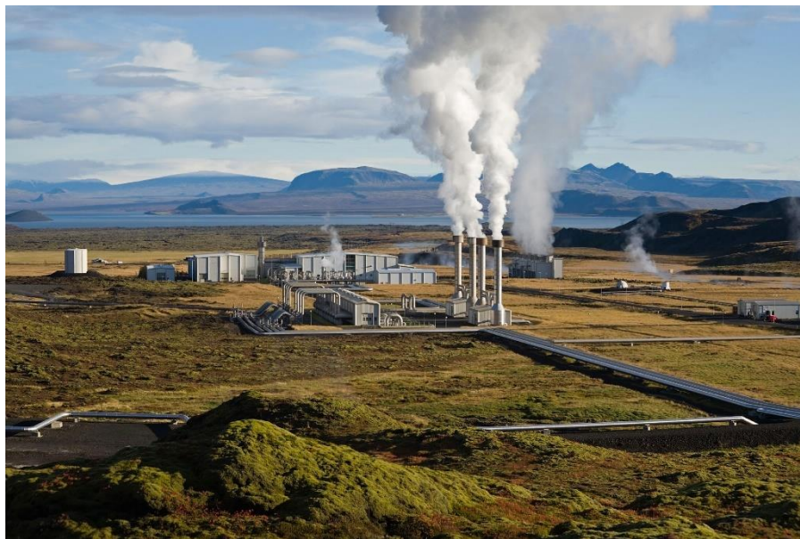
Figure 29. General view of a geothermal power plant.
