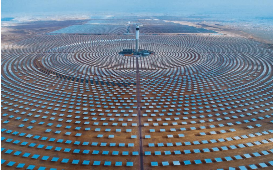
Figure 14. General view of a solar power tower plant
