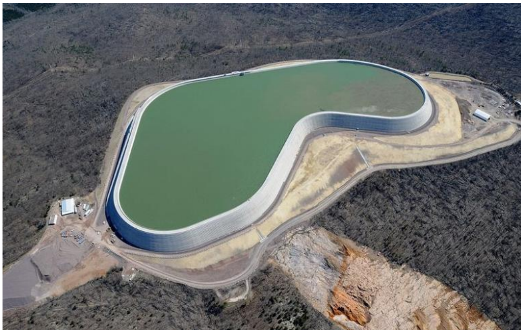
Figure 30. View of the PSHPP reservoir Calculation of energy stored by PSHPP
