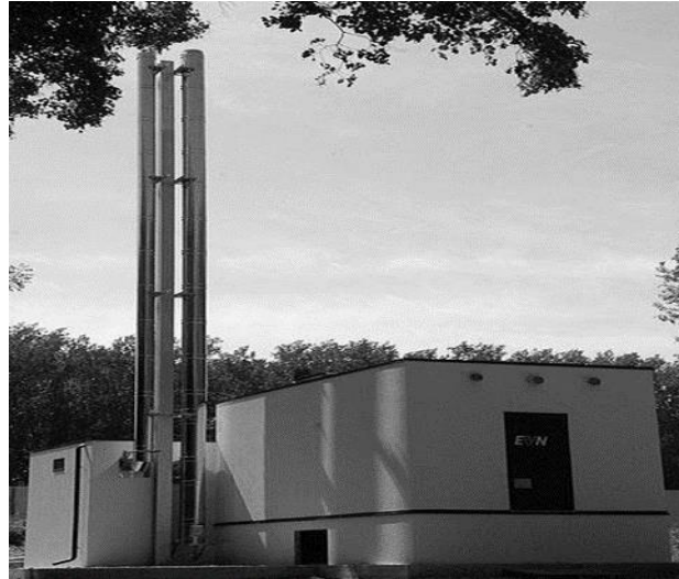
Figure 26. General view of a 1000 kW biomass-powered heating plant (Austria) [1].
