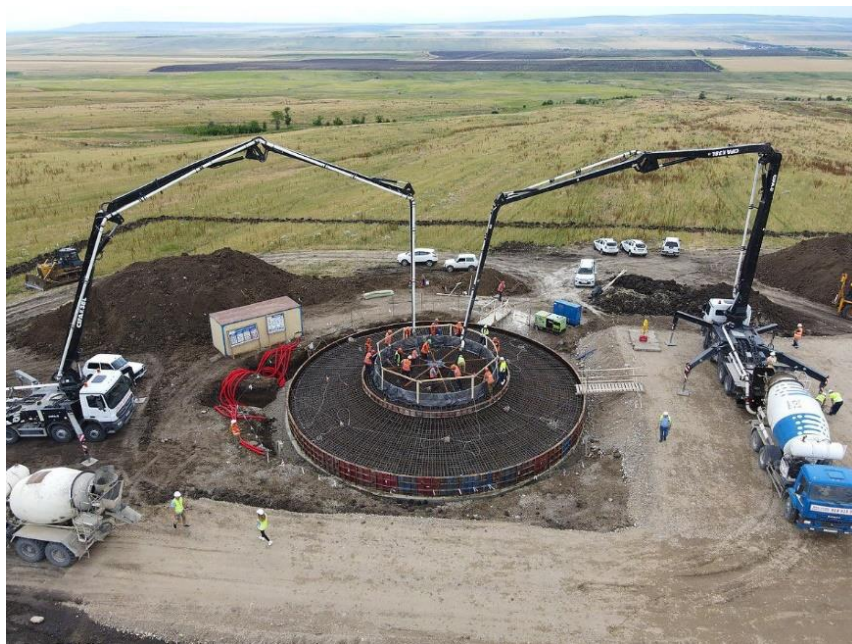
5.11-rasm. ShESning birinchi poydevorini quyish jarayoni.
