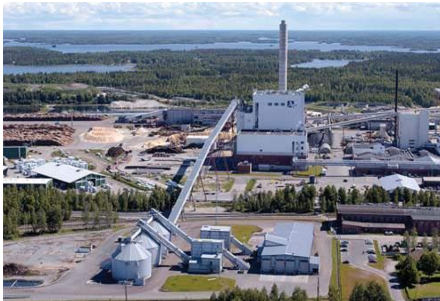
Figure 7.1. View of the world's largest biomass-fired power plant.
