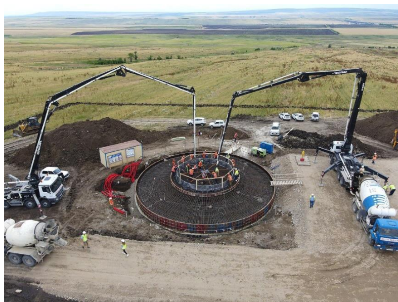
Figure 5.10. Construction process of the first wind power plant foundation.
