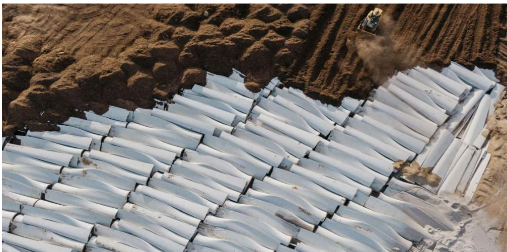
Figure 5.18. Landfilling process of wind turbine blades.
