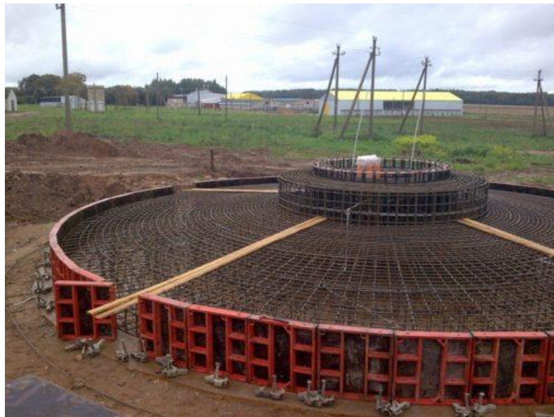
Figure 5.9. Wind power plant foundation pouring process.
