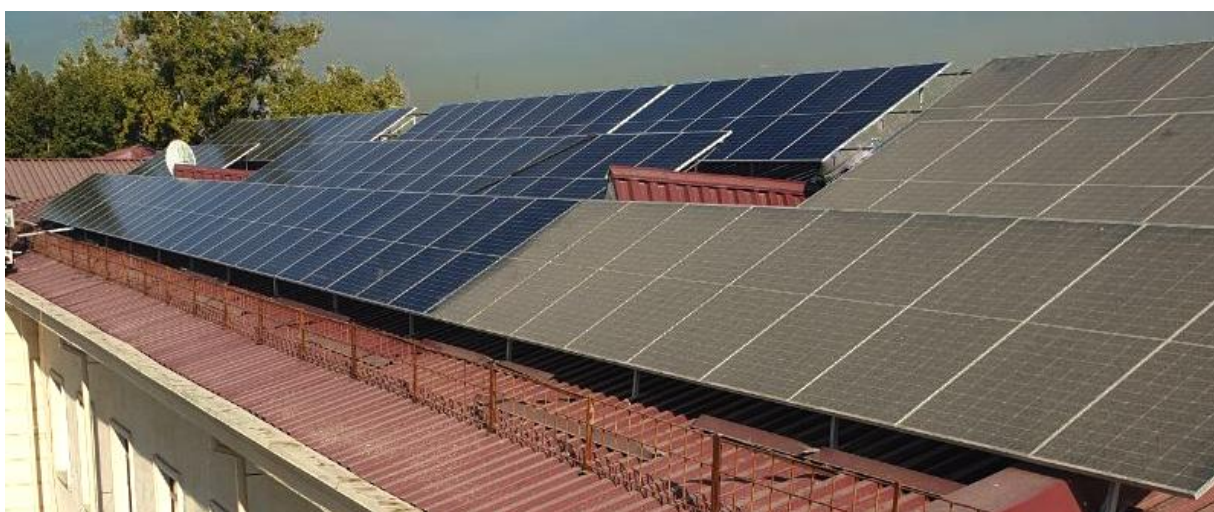
Figure 2.27. Photovoltaic modules before and after cleaning.
