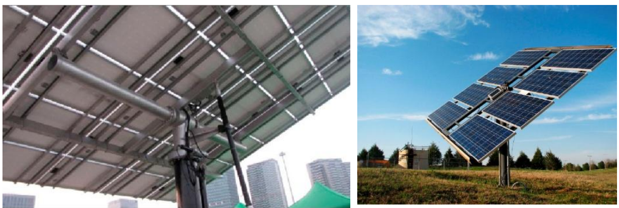
Figure 3.21 Two-axis tracker solar power station
